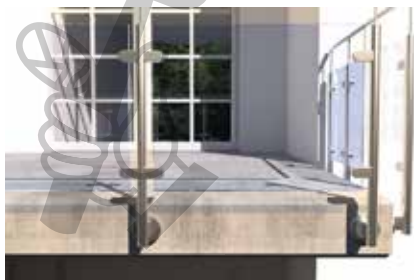
Railing anchorages
