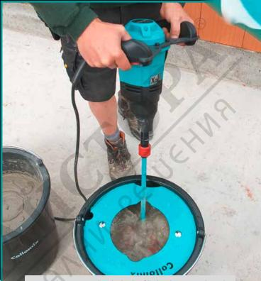
Immerse the mixing tool in the bucket filled with water and run the mixer for a short time, clean!
