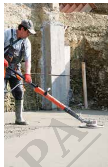
Levelling fresh concrete
